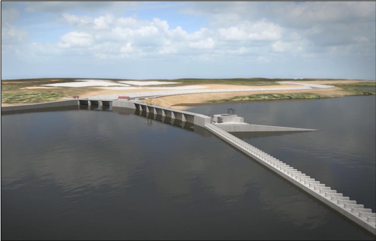
Figure 2.3: View of the Nachtigal main dam
