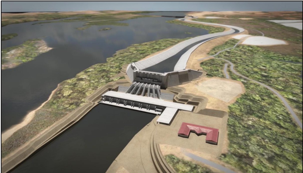
Figure 2.4: View of the Nachtigal Power House
