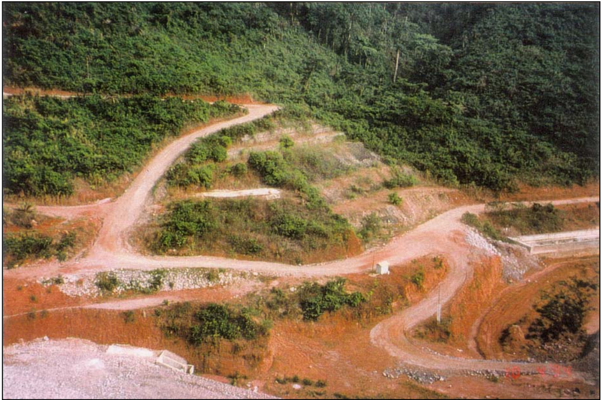
Figure H.5.3-3: Earth Moving Activities near the Dam Site.
