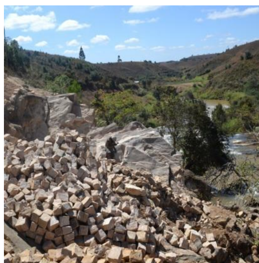
Meshing of rubble near the weir (S17°46'53.39 E48°5'38,99)
