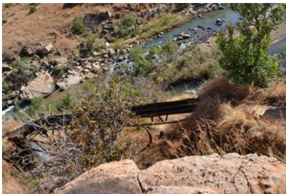
Suspended irrigation canal
