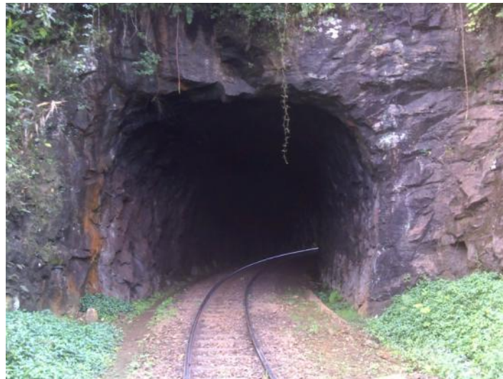
Figure 16. Existing tunnel for the railway adjacent to the site
