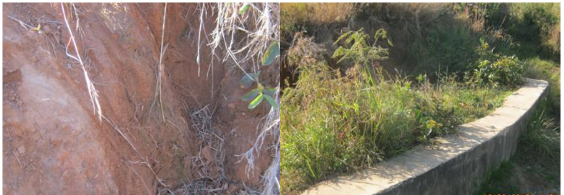
Figure 11. Right bank support of the existing weir
