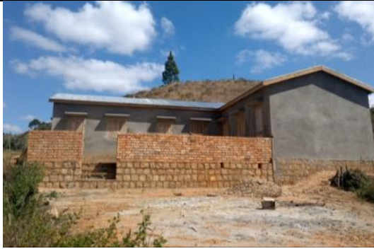
Technical-administrative building (work in progress)
