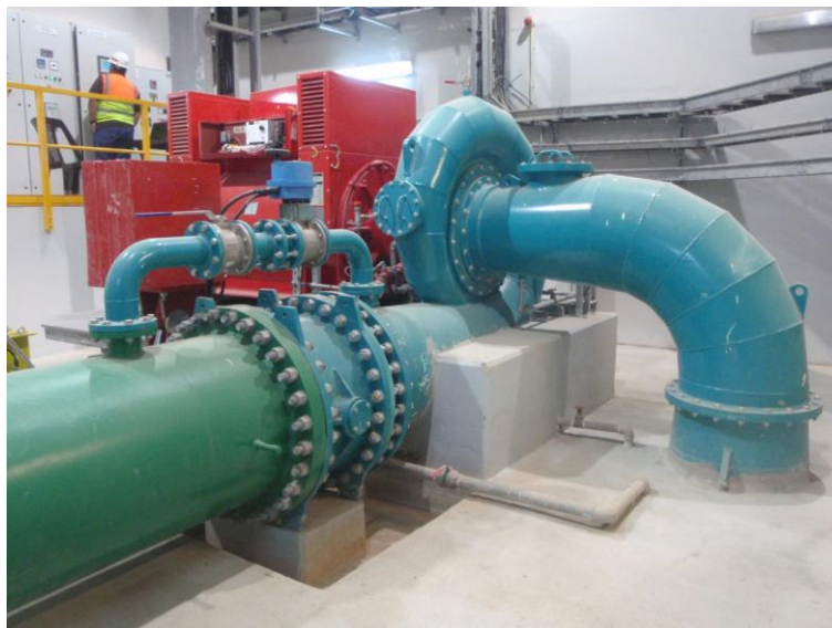
Figure 14 Example of a horizontal axis Francis turbine
