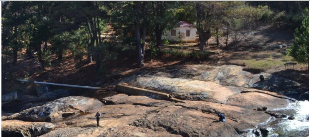
Catchment near the bridge, for the hydropower plant of the forest station S18°9'27.42" E47°12'36.86"
