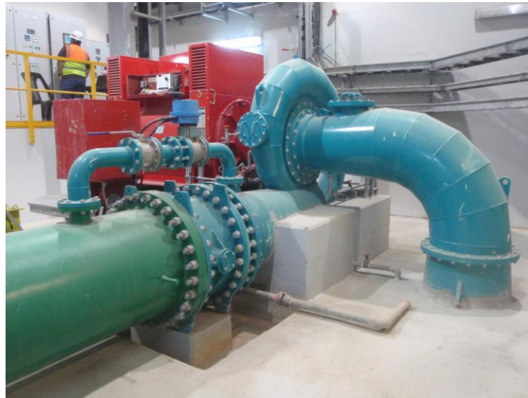
Figure 13 Example of a horizontal axis Francis Turbine
