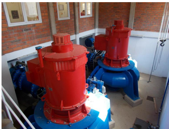
Figure 18. Example of 2 set with vertical axis
