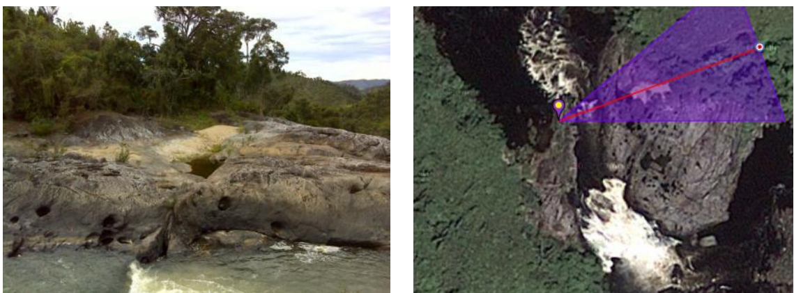
Figure 14. Partial view of the proposed weir site.
