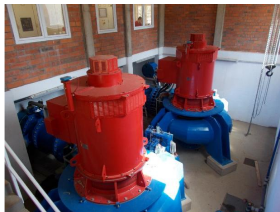
Figure 15. Example of two vertical axis Francis units
