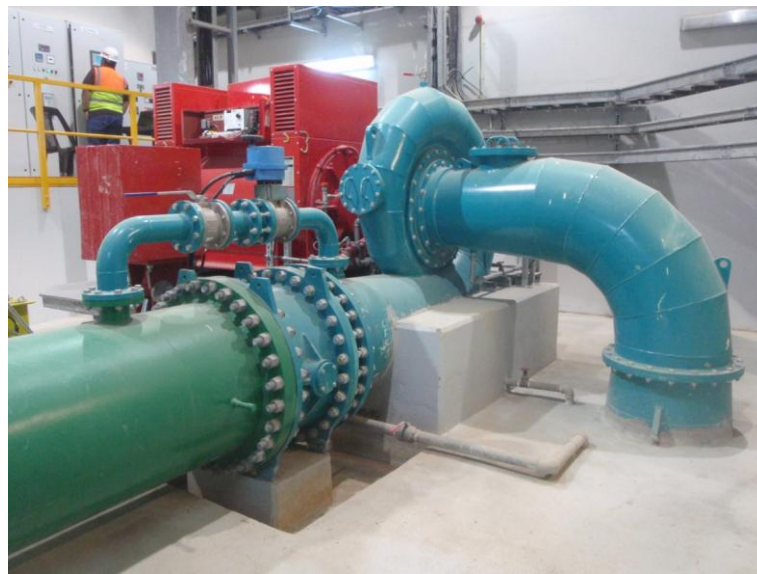
Figure 20 Example of a horizontal axis Francis Turbine
