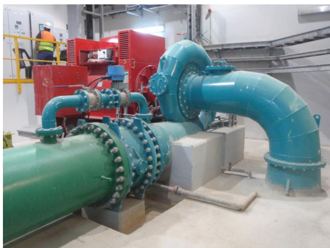
Figure 15 Example of a horizontal axis Francis unit
