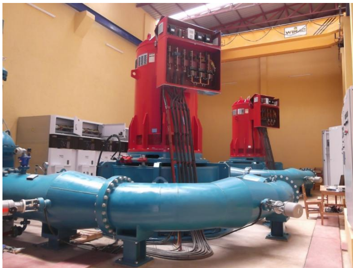
Figure 18 : Example of a 5-injectors Pelton turbine
