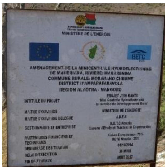
Info panel about the on-going mini hydroelectric plant
