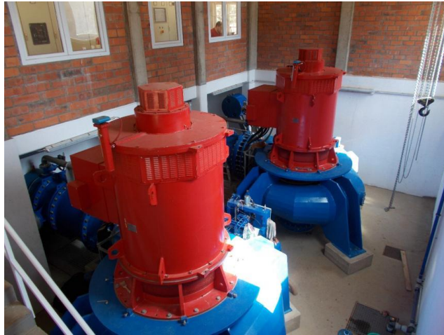
Figure 15. Example of a vertical axis Francis Turbine
