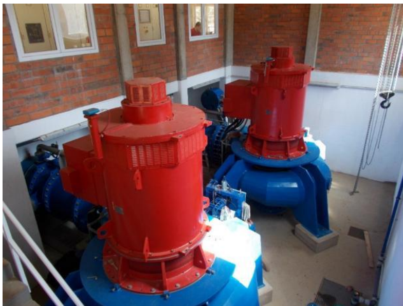
Figure 15 : Example of two vertical axis Francis units
