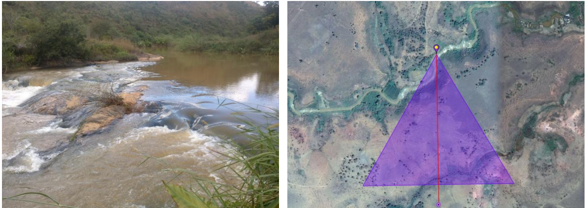
Figure 4. View of the proposed location of the weir.
