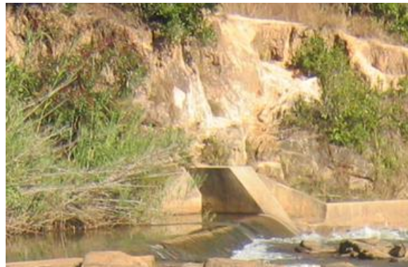
Figure 12. Right bank support of the existing weir
