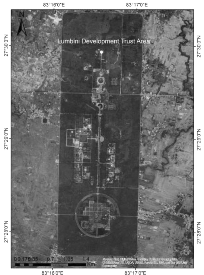
Figure 1: Aerial view of Lumbini Development Trust Area
