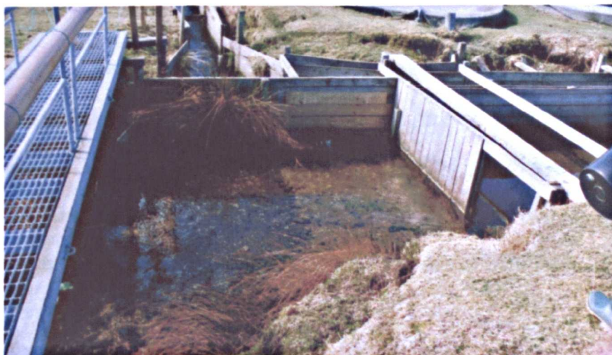
Figure 2.1.D Settlement pond at the end of the outflow canal of the salmon hatchery.
