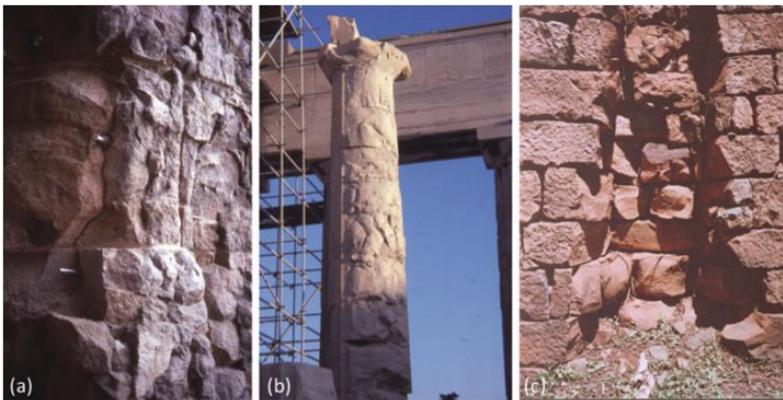
Figure I-9. Examples of effects promoted by historic fires in stone-built structures. Granite pillars, Brazil (a), marble columns, Greece (b), church wall constructed with argillaceous sandstone, Argentina (c) (Siegesmund and Snethlage, 2011).
