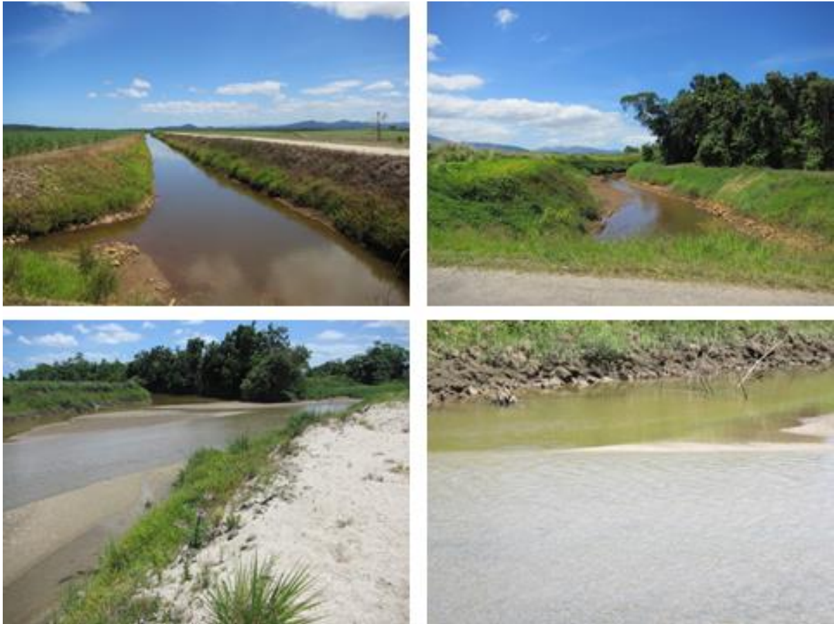
Figure 2.3.13: Above – The main Babinda Swamp Drain channel. A network of smaller drains connects with the main channel to form the Babinda Swamp Drain program. Note the oxidised stain to the water. The drainage program is managed by the Babinda Swamp Drainage Board. Below left – The main drainage channel joins Babinda Creek approximately 200m from its junction with the Russell River. Below right – Water exiting the Babinda Swamp Drain (top of picture) has a significantly different appearance to the very clear water of Babinda Creek (bottom of picture)
