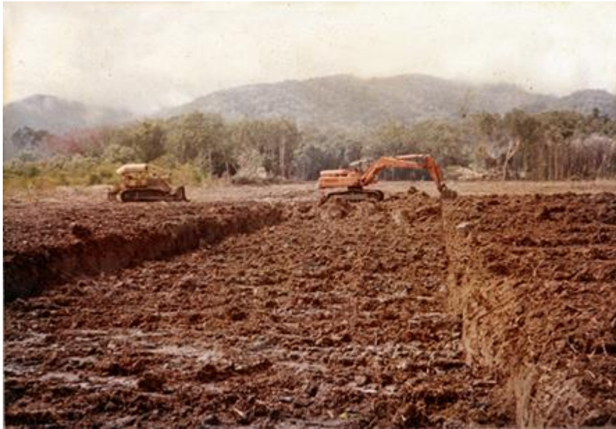
Figure 3.1.1: Cane drainage channel under construction in the 1970s (image DEHP)
