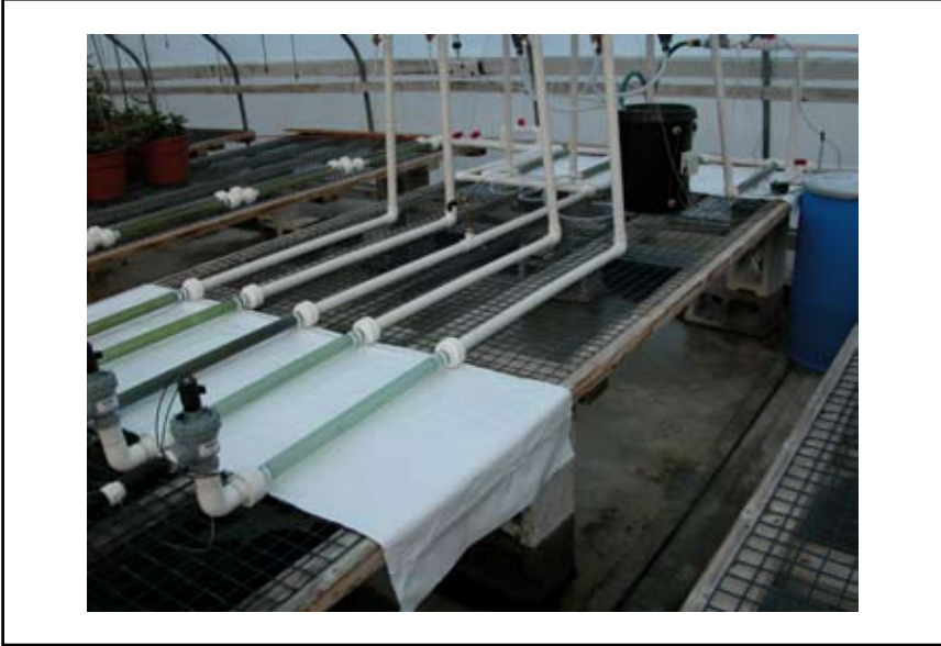
Figure 9. Clear sections of PVC installed to view algae and biofilm development.
