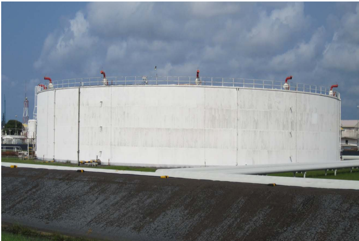
Figure 3: Wash Tank for Primary Oil Separation and Removal
