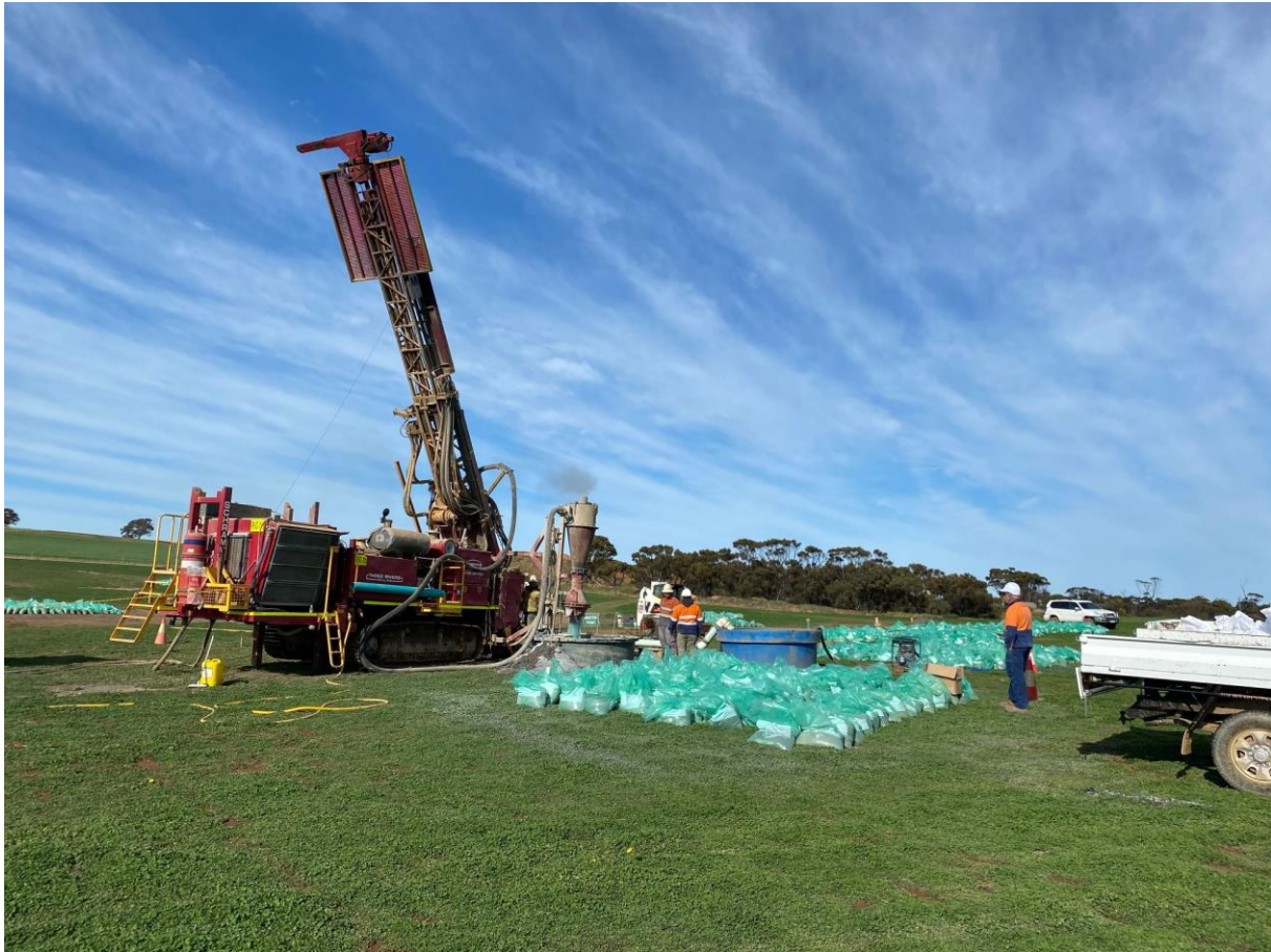
Figure 12: Groundwater containment system
