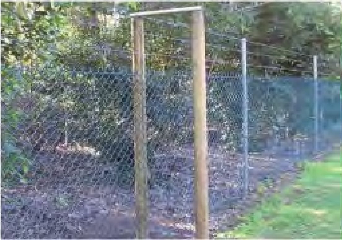
Plate 9. Example of a Koala bridge to provide connectivity across a fenced barrier to movement (DES, 2020).
