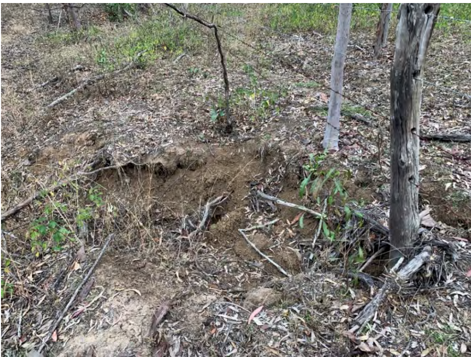
Plate 3. Minor erosion and scouring identified within the eastern section of the Property boundary.
