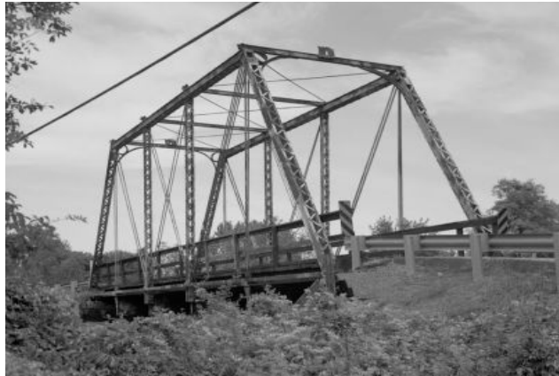
Figure 3-14: Photograph of the iron truss bridge, the last remaining one in the county. Source: CHG
