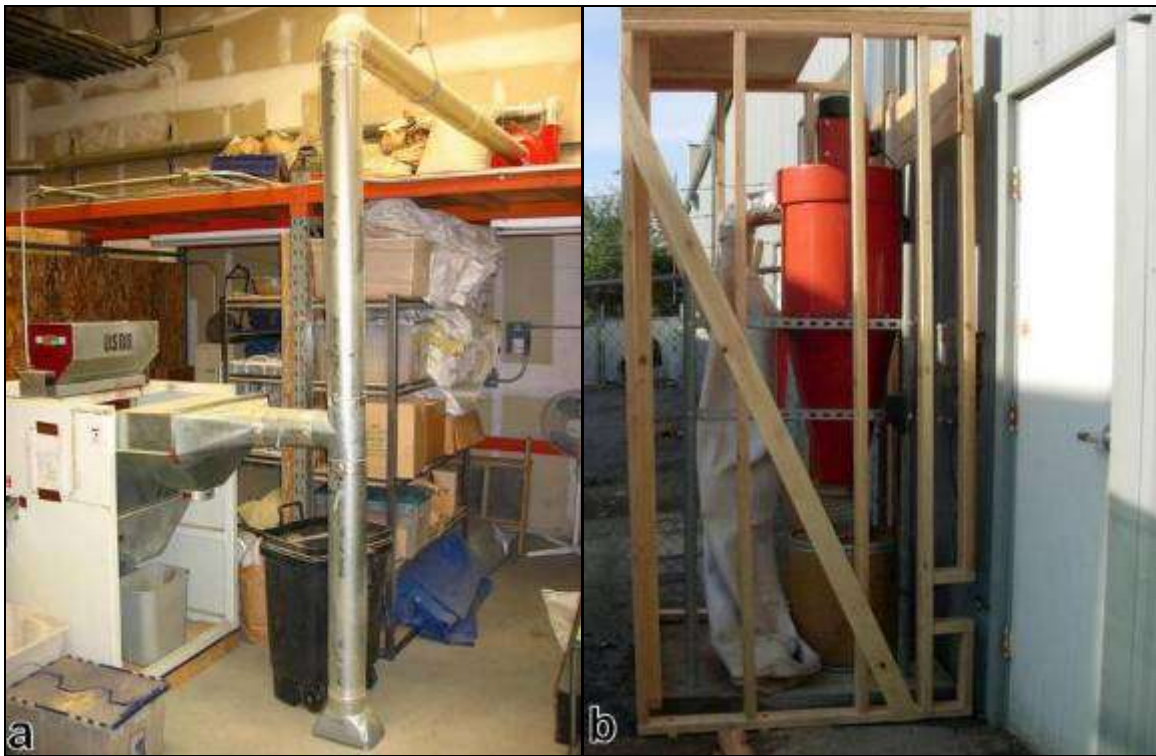
Figure 26. Dust removal system. a. The dust removal system included a hood that attached directly to the Clipper Eclipse seed cleaning equipment. The dust moved through the ductwork and was collected in a receptacle located outside of the building. b. The dust collection vacuum and receptacle were stored outside of the building due to the level of noise that the vacuum produced.
