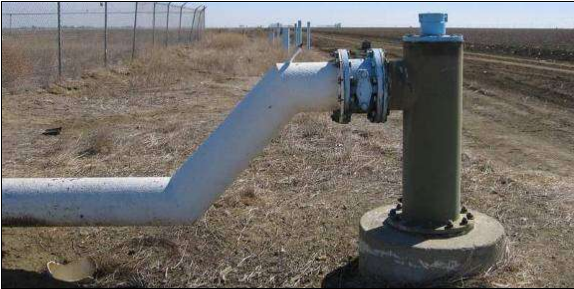
Figure 10. The nursery site is located within Westlands Water District. This “turnout” is part of the Westlands water distribution system. To irrigate the nursery, irrigation pipe was connected to the turnout and a water order was placed with Westlands Water District.
