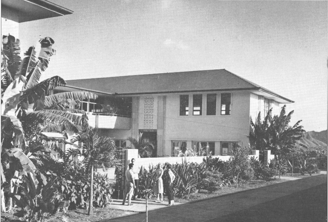
Hemenway Hall, union building.
