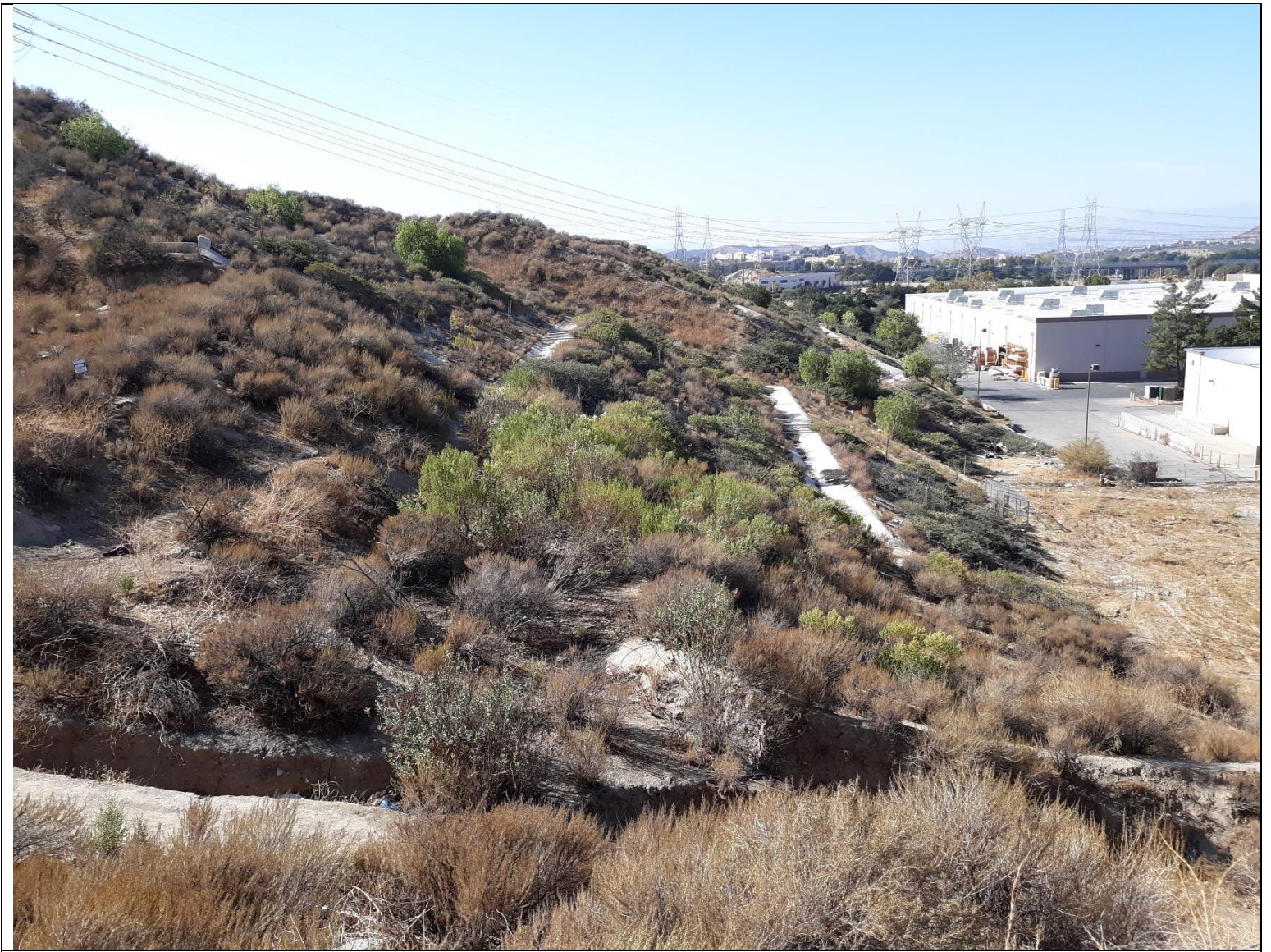
Lots 1 & 4, manufactured slopes on of Lot 1. Viewing west. Feature 3 (headcut erosion gully) in foreground.
