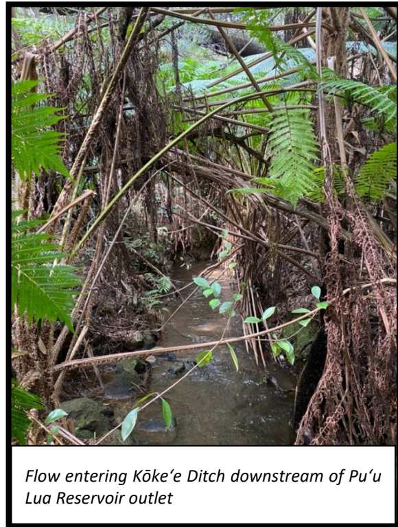
Pu'u Lua Reservoir outlet works
