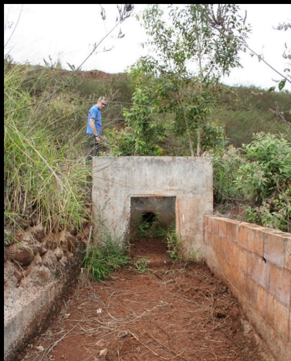
Existing downstream outlet at Pu'u 'Ōpae Reservoir and connection to downstream irrigation
