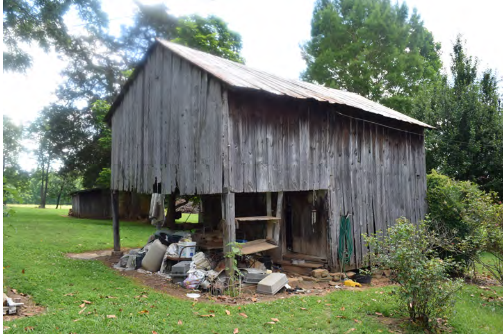
Well house and shed (background) view to the northeast
