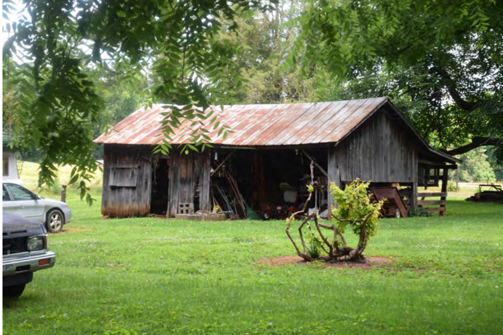
Garage/shop, view to the north
