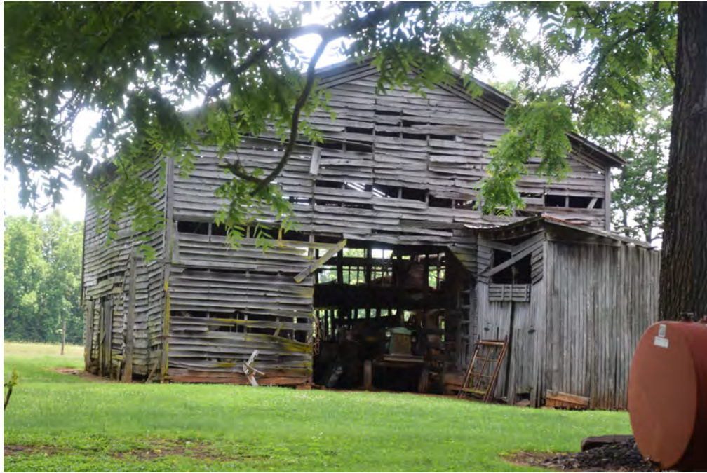
Barn, view to the northeast
