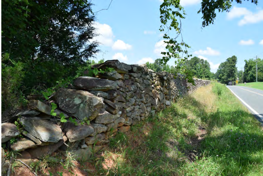
Rock wall, view to the northeast
