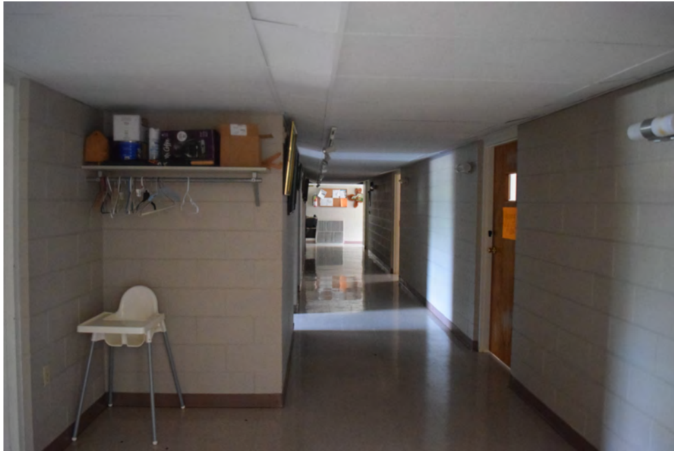
Lower level hallway, view to the north-northeast
