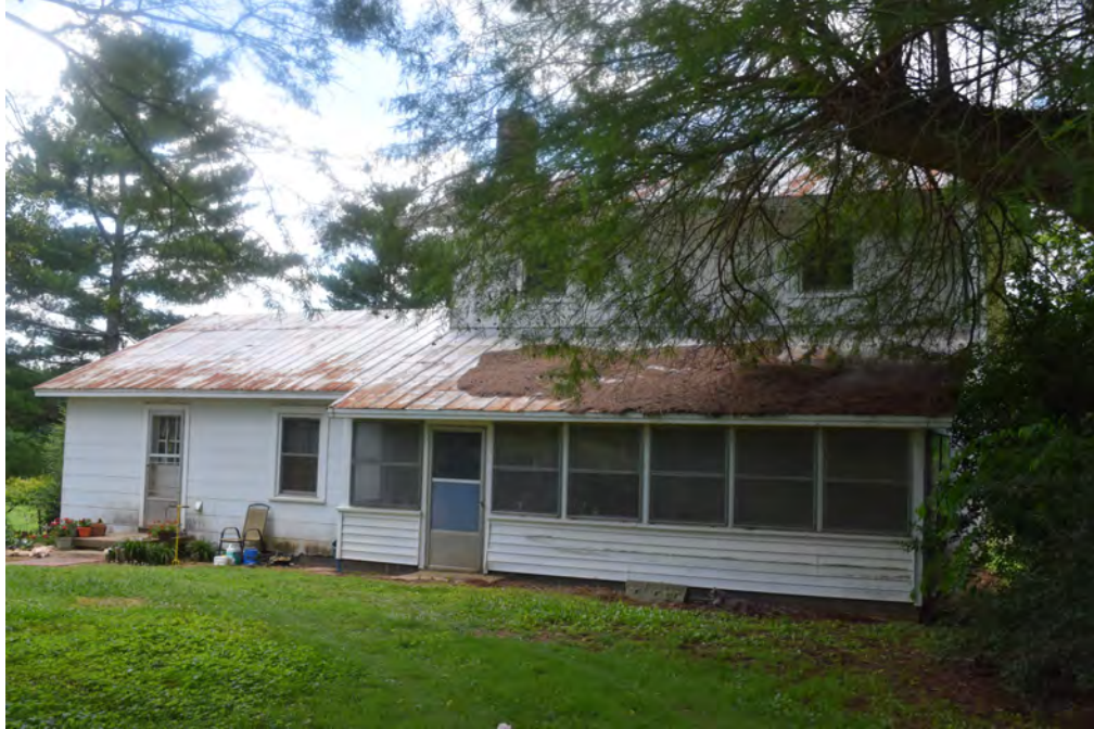
Rear elevation, view to the south-southwest
