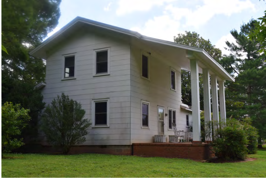
West façade, view to the east
