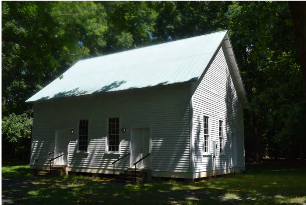
West Grove Meeting House, view to the north
