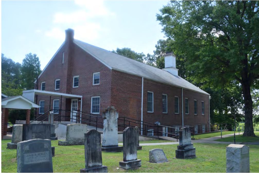
North corner of the meeting house, view to the south
