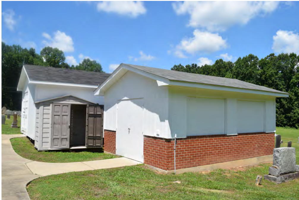
Pot house (foreground) and storage building, view to the northwest
