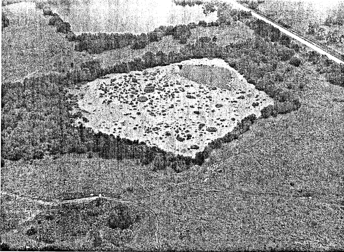
Figure 7. Aerial view of the Coronet Minerals, Inc., inactive phosphate pit in Coronet Junction, Hillsborough County, Florida.
