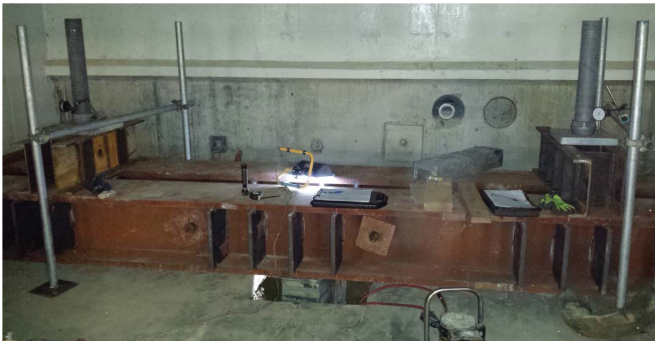
Figure 4: Structural frame and vertical anchors supporting Test 2. Plate is located within the pit below the cut floor slab in the centre of the photograph.
