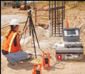
Pile Integrity/CSL Testing
