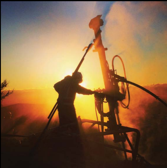
Gareth Hallam - Abseil Access drilling in perfect conditions
