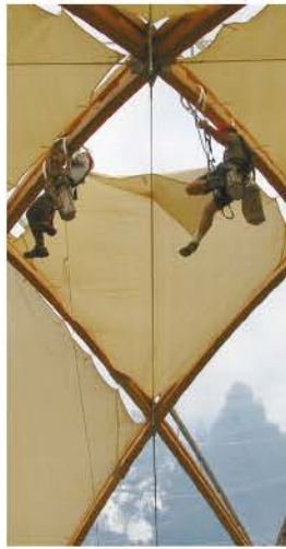
REMOTE MAINTENANCE & INSPECTION
