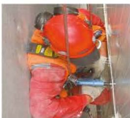
CONFINED SPACE ACCESS
