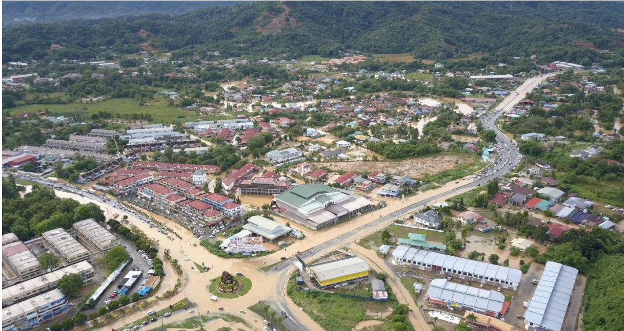
Figure 9. The precipitation shock induced by the Ewiniar typhoon has caused flood in Donggongon, Penampang, a suburban district of Kota Kinabalu city that is located in the foothills of Babagon. This image was recorded on 1st June 2018.
