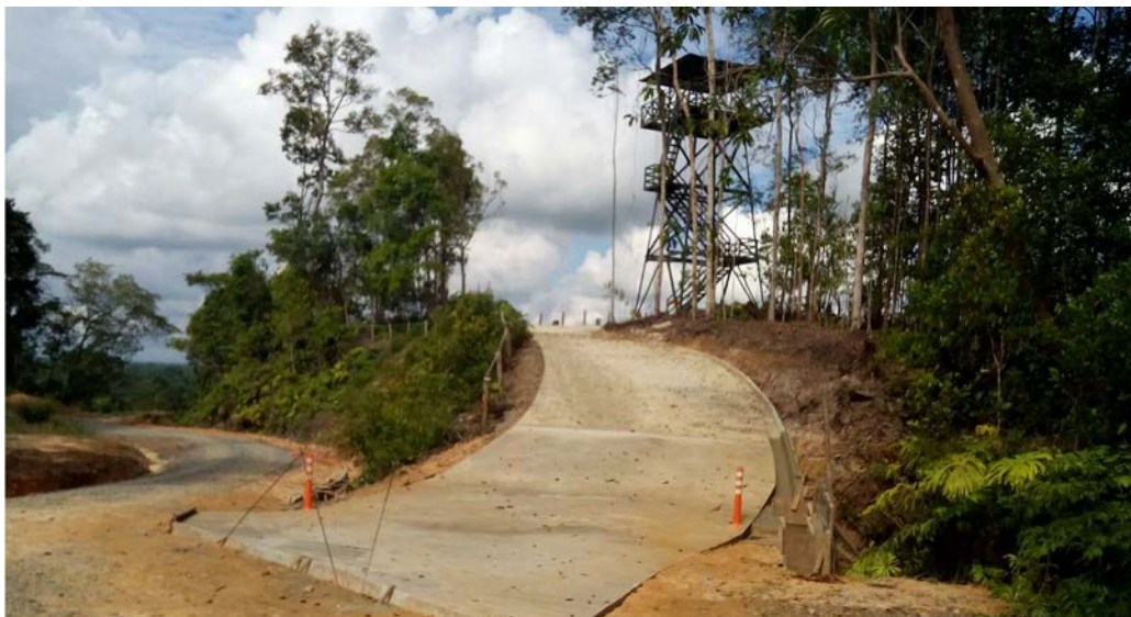
Photo 3: The fire tower located close to the Fidelis Peak in Compartment #5.
