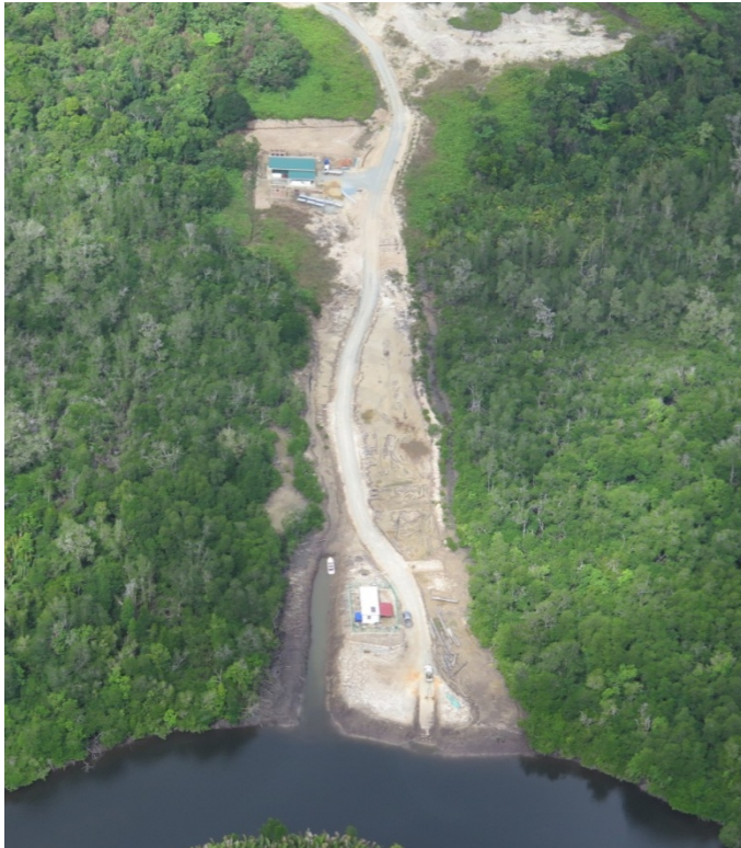
Photo 2: (left) Sg. Timbang Jetty in Compartment #4. The helicopter landing pad can be seen in the upper right corner.
