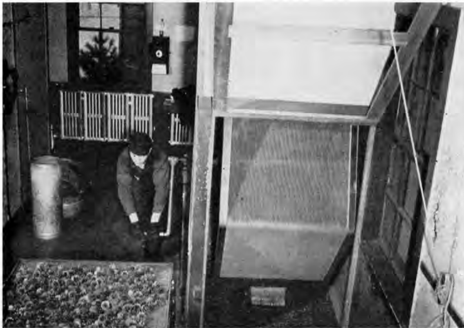
FIGURE 3.—Cone shaker.
