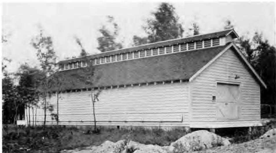
FIGURE 1.—This cone storage shed is 30 by 70 feet and will hold 2,300 bushels of red pine cones on trays. (Chittenden Nursery, Wellston, Mich.)
