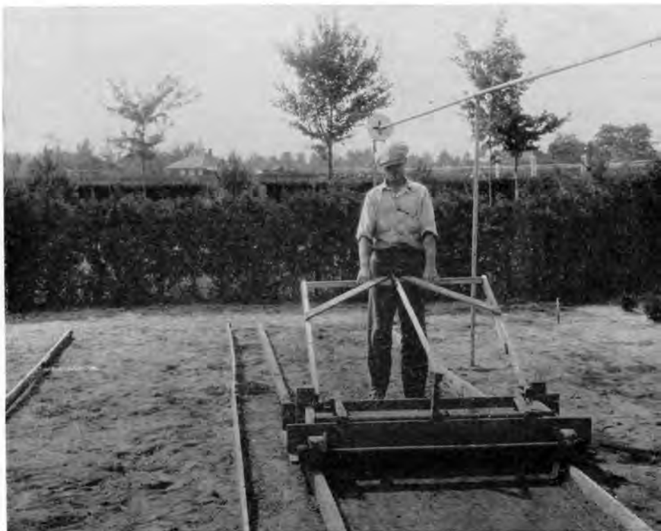
FIGURE 34.—A hand-drawn bed leveler equally well adapted for drill- or broadcast-sown beds.
