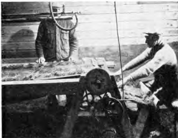
FIGURE 55.—Culling or grading table with endless belt.
