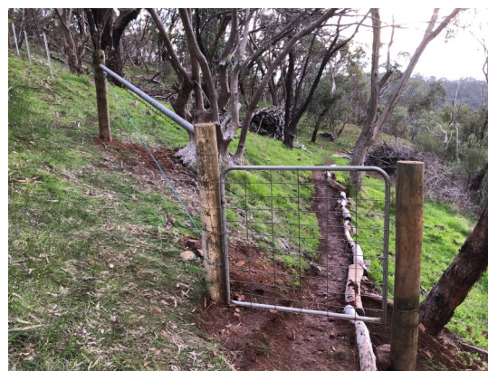
Rebuilt Stone Reserve fence with new gate on walking trail
