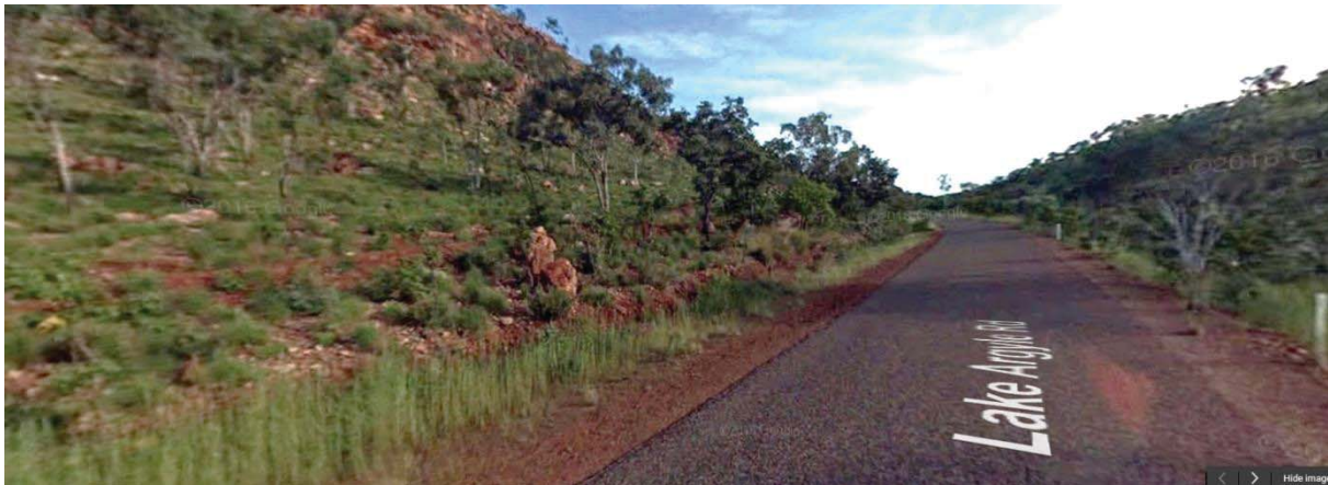
Figure 1: Representation of the existing Lake Argyle Road within the rocky outcrop area
