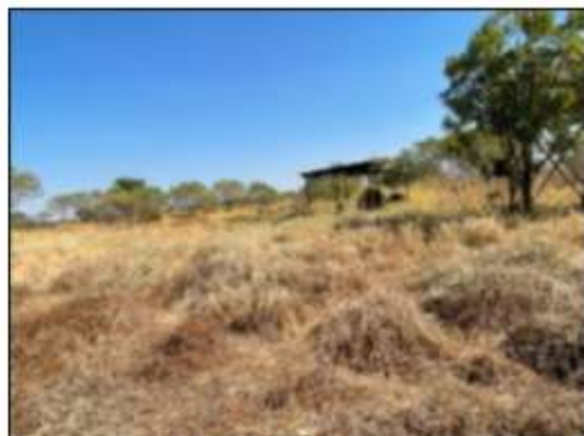
Old pump shed at waypoint KCC10
