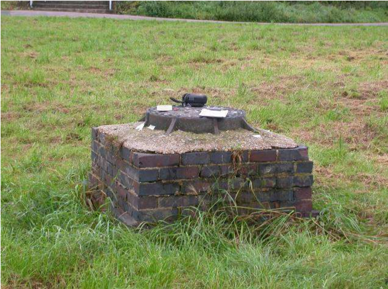
Figure 6. Concrete surround of manhole cover at TL4718.5923.
