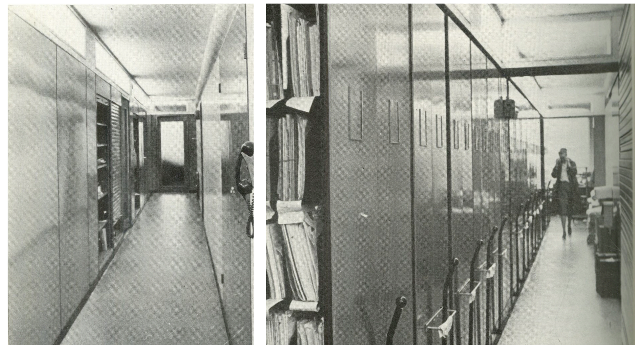
VIEW S OF INTEGRATED LIGHTING SYSTEM IN CORRIDORS
