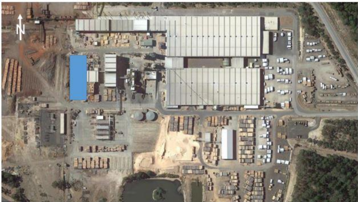
Figure 3-1: Bell Bay timber mill site layout – including proposed WPC Facility building (shaded blue)
