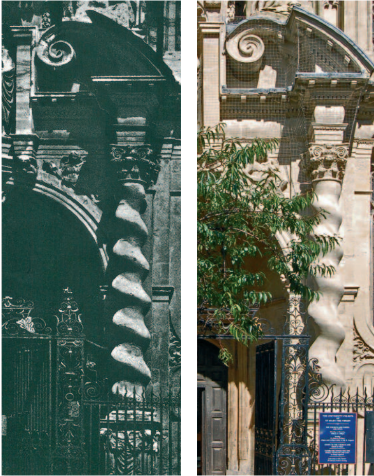
Fig. 7. The right hand Solomonic column in St Mary's a photograph of 2014 compared with one c.1960. The old image clearly shows equal dimensions between the crests (in adherence to Vignola's method) in the modern image the dimensions are markedly greater lower down the shaft than they are at the top.
