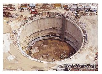
Fig.2. Excavation within the temporary cofferdam
