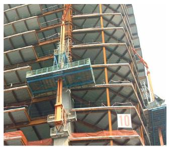
Fig.4. Column Climbform System
