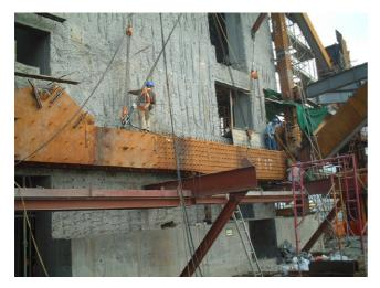
Fig. 7. Retro-installation of steel outrigger within the core wall
