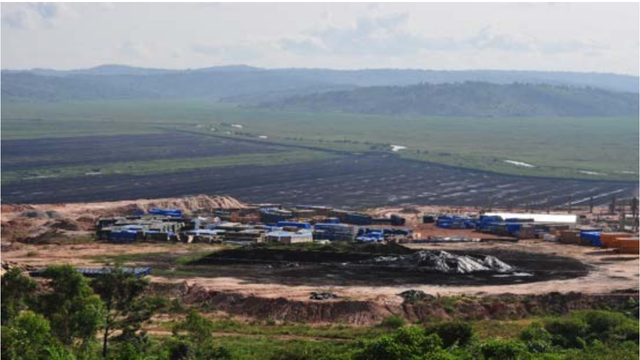
Figure 3.14. Peat-powered electricity plant in Gisagara, Rwanda. Photo: Hans Joosten
