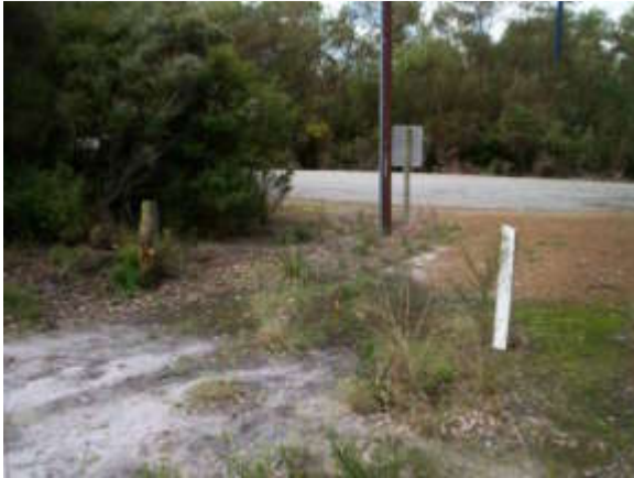
Damage to fire access track barrier at Lake View Place
