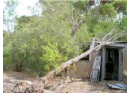
Derelict shed below Minsterly Road
