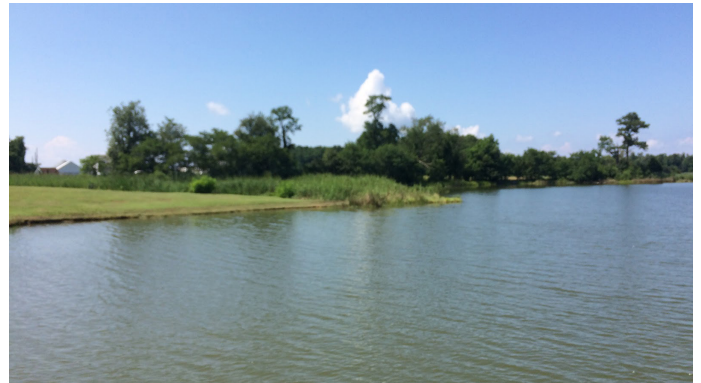
Timber bulkhead to the left of on-shore stone. (Rebecca Swerida)
