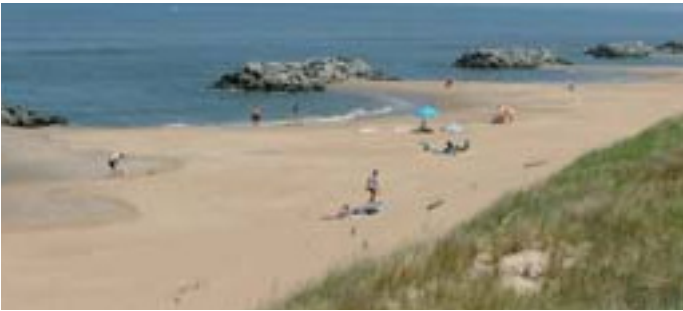
Large off-shore stone breakwaters structures are sometimes connected to shore by tombolos of sand at very low tides. (Virginia Institute of Marine Science)
