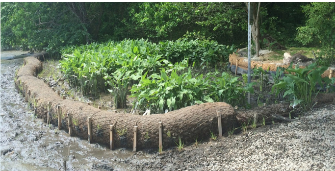
A newly placed coir log protecting a freshwater marsh. (MD DNR)
