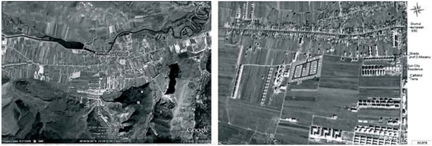
Figure 1. Studied residential development background
