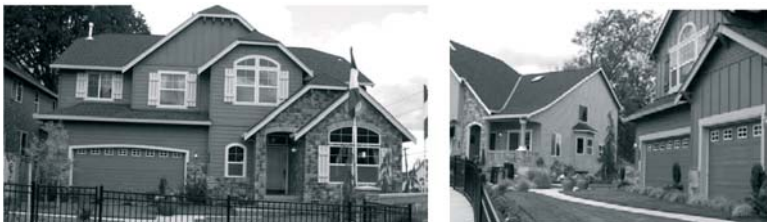
Figure 2. Example of reducing the visual impact of garages on the site appearance [8]
