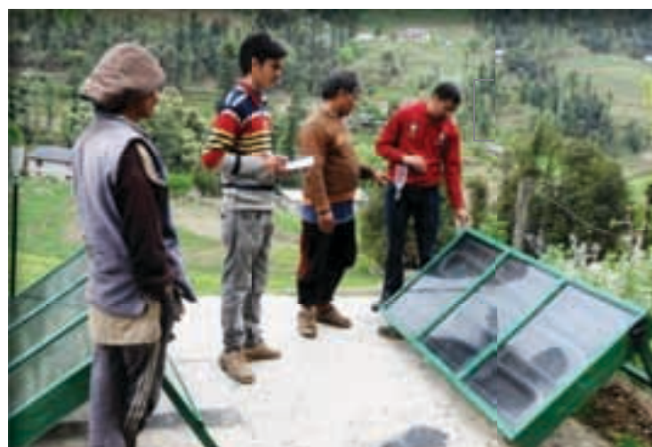
Installation of solar water heating systems at Mandi (H.P.)
