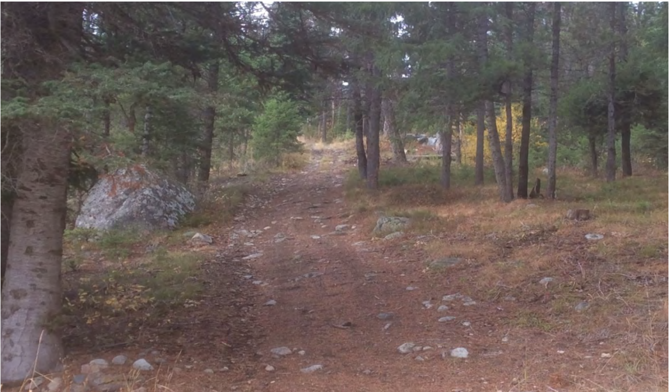
12' wide x 1321.56' long right-of-way for the buried 4" penstock and steep ATV access trail to the diversion
