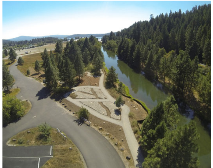
Garden overview immediately post-construction, August 2014. Drone operated by Dan Lyden.
