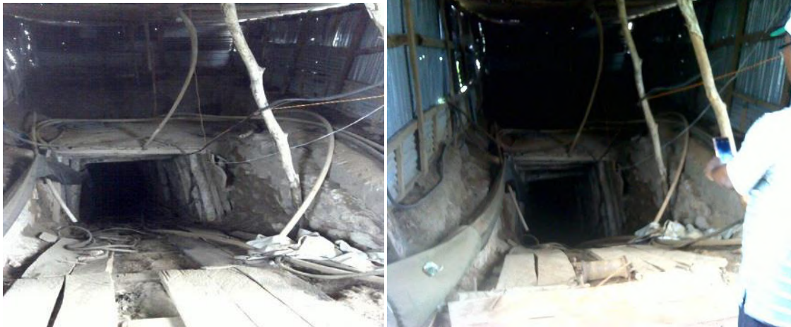
Plate.1: Underground mining Tunnel at Jukun Village in Karim Lamido LGA
