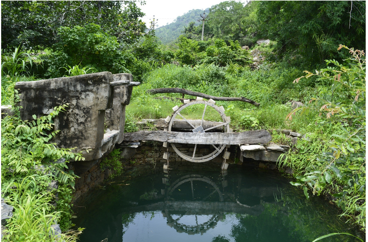
Figure 6: A Persian well in catchment area of Banas river
