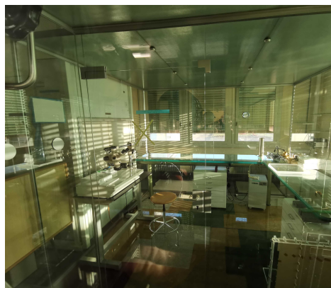
R-006 clean room
