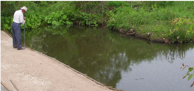
The dipping pond on completion
