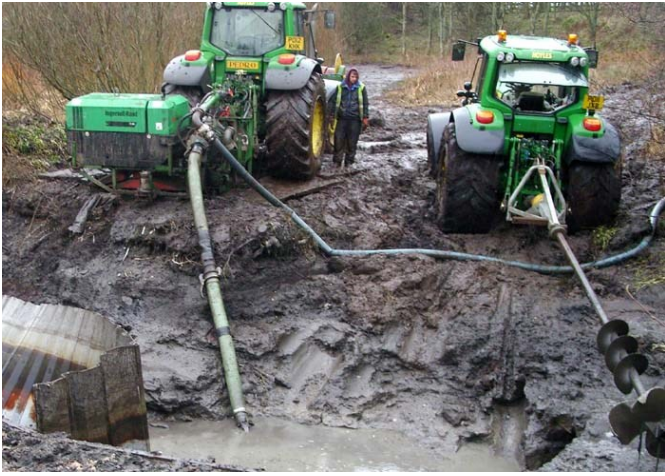
Dredging of the dipping pond
