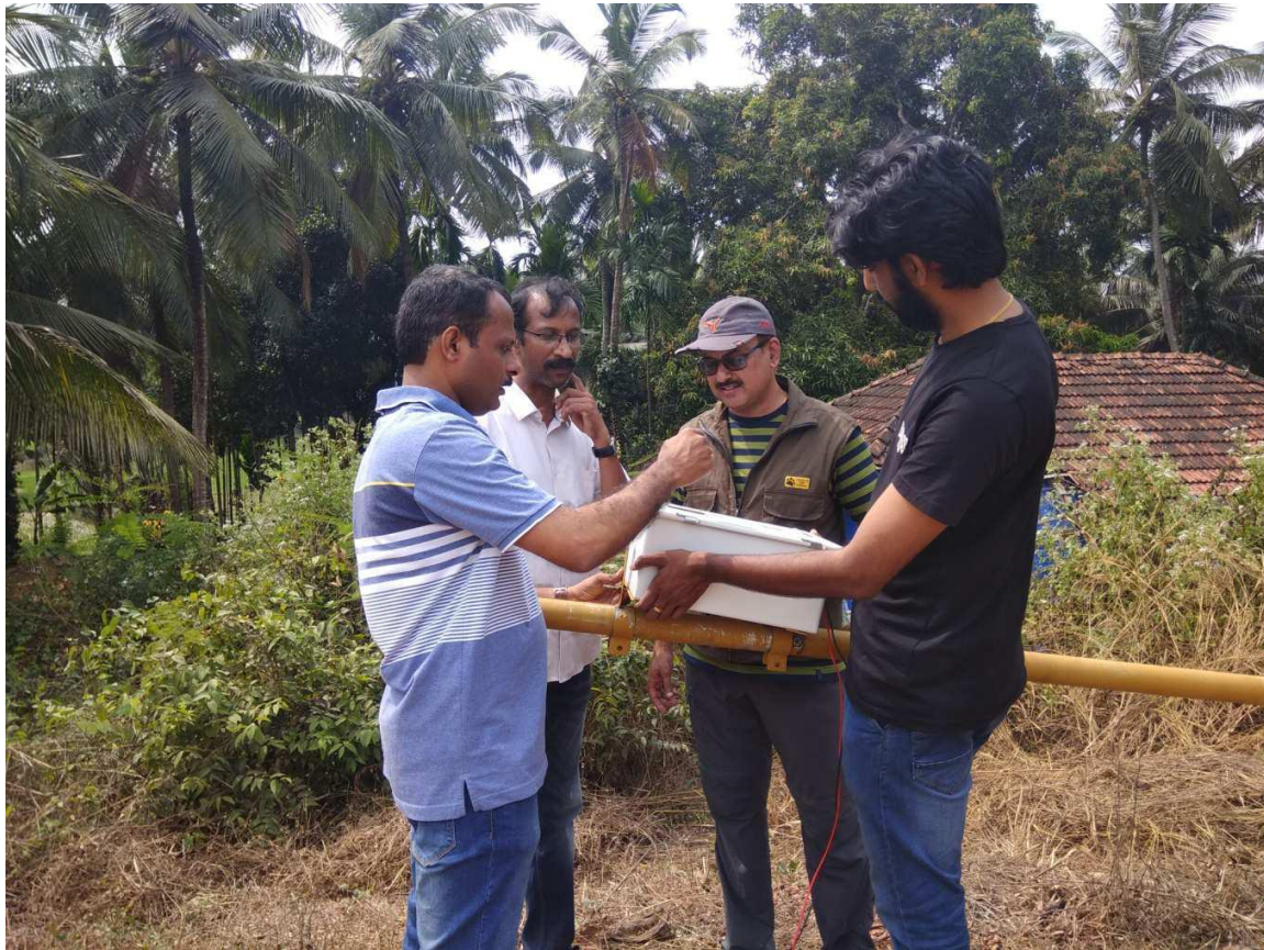
System Installation at Palakkad
