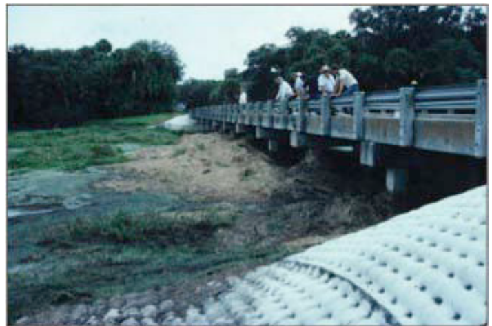
Figure 16. Submersed plants piling up on a bridge in South Florida. Credits: Ken Langeland, UF/IFAS Extension
