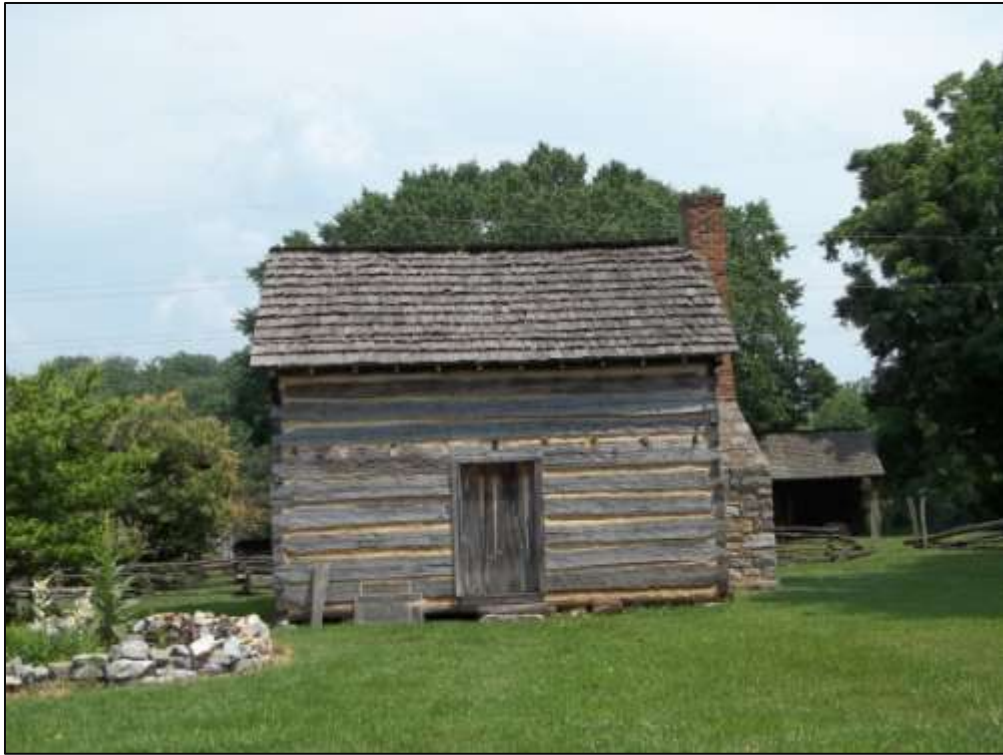
Figure 4. Rear of George Haynes Slave Cabin. Photograph by author.
