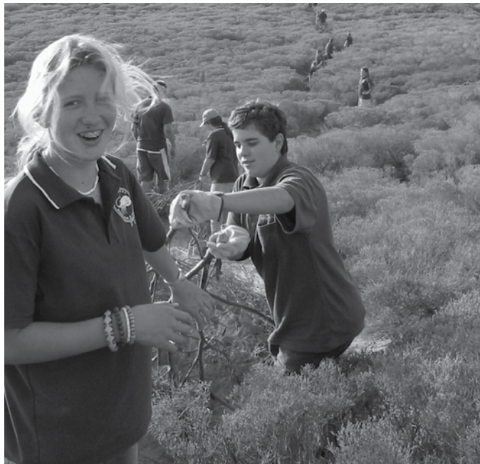
Bushrangers from Kalbarri District High School work on walk trail construction between Natural Bridge and Island Rock. Photo – Sue Hancock (DPaW)
