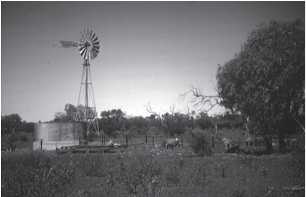
Natural water is scarce in much of the rangeland but pastoralists provide troughs for stock such as this one south of Wiluna which is supplied by a windmill. Checking on the windmills is an essential job on the stations, particularly in summer.
