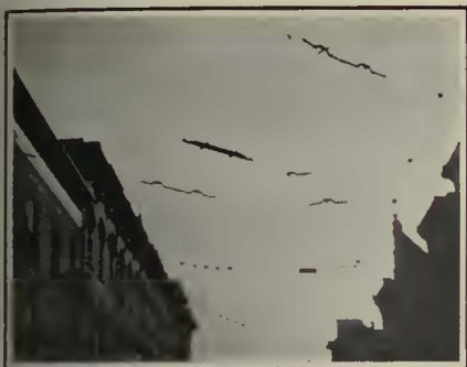
Overhead Construction Used with Trackless Trolleys. At Left, on Remsen Street, Where Trolley Buses Parallel Existing Electric Line. Center, Y Construction at Columbia Street Terminal. At Right, Overhead at Manor Avenue Terminal
