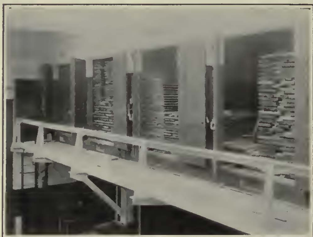
The Dry Lumber Storage Has Six Rooms, Each 16 Ft. Square, and Heated by Steam Coils
