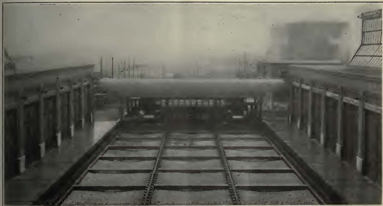
The Transferway Constitutes the Main Axis for the New Boston Shop—The Paint Shop Is on the Left and the Kiln Building and Wood Mill on the Right
