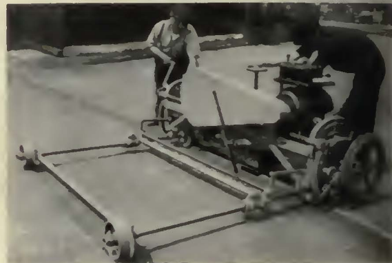
"Vulcan" Rail Joint Grinder
