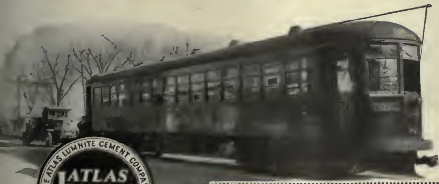
LUMNITE was used for this trolley roadbed in Hudson, N. Y. Concrete was placed on the morning of October 25, 1924, and 32-ton trolley cars were put in operation on the new road the morning of October 26th—only 26 hours after completion with LUMNITE.
