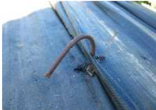
Photograph 4.- Fixing the two black net pieces over the center of the ridge
