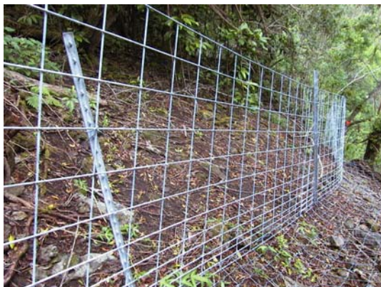
52" hog panels and ground skirt
