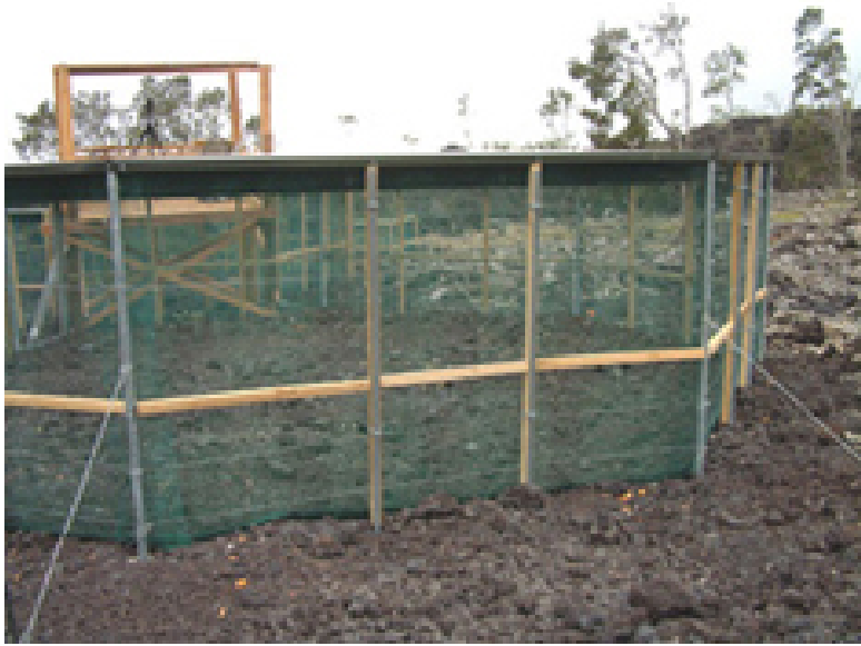
Excluder fence demonstration project on the Big Island done to assess effectiveness on uneven lava substrate.
