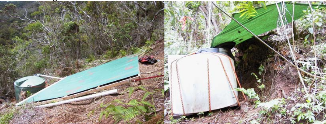
A large 1500 gallon tank feeds a smaller 250 gallon tank which is also rigged for catchment.
