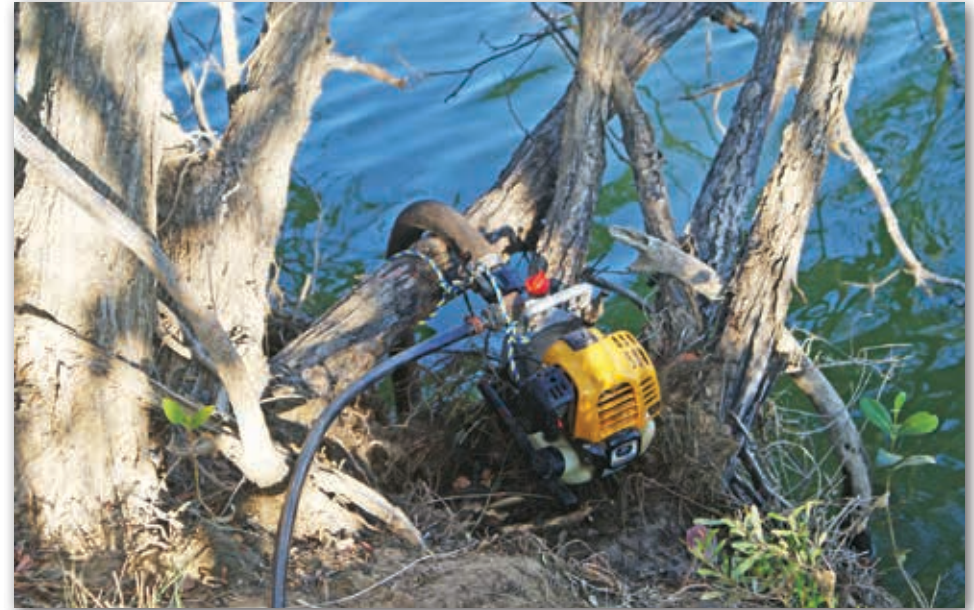
Pumping water straight from the creek.
